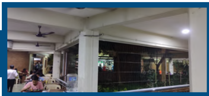
Monkey Proofing work at Quark building
