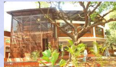
MONKEY PROOFING FOR QUARK BUILDING
