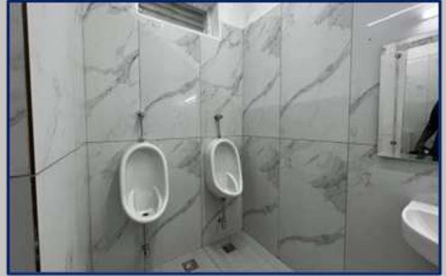
Rest rooms (Ground floor – Front Wing)
