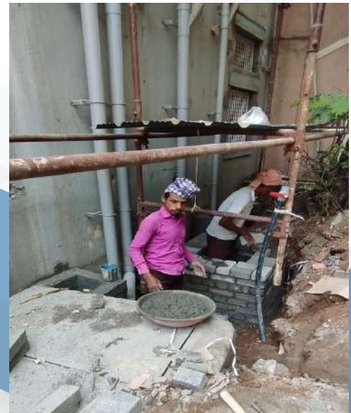
External Chamber Construction
