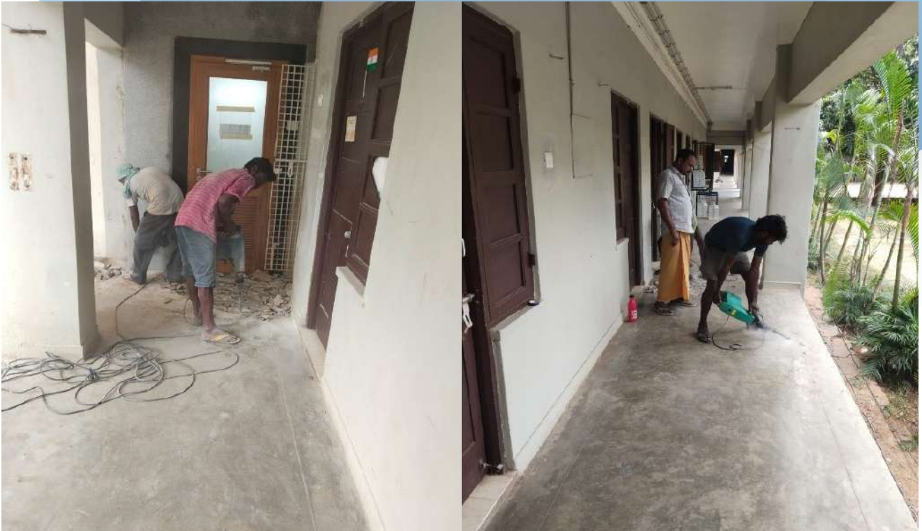
Corridor Demolition Work
