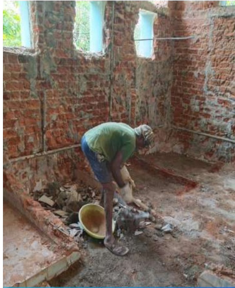
Debris Cleaning Work
