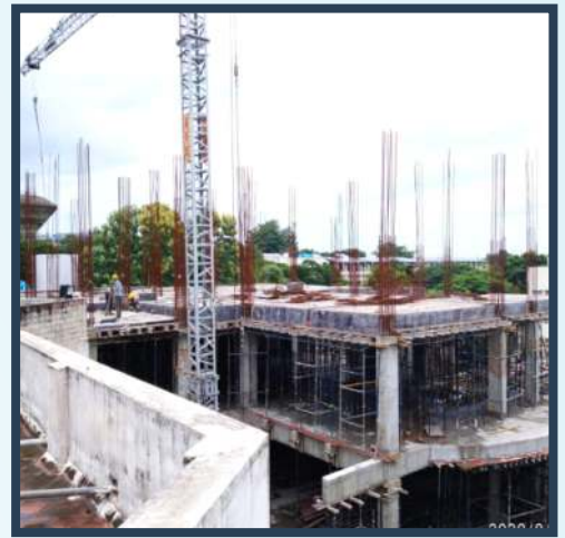
3rd Floor Balance 70% Slab Shuttering
