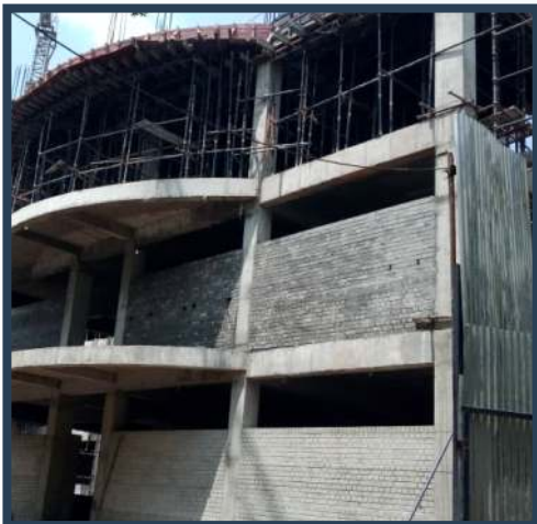
Structural work - G+2 completed
