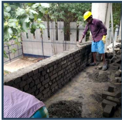
1st Floor Block work in progress
