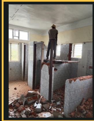
Breaking the restroom partitions
