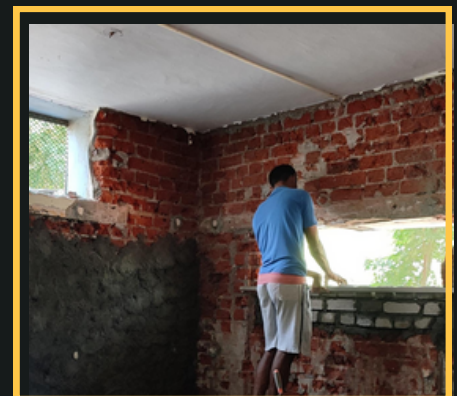
Brickwork in restroom
