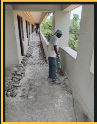
Breaking the cement flooring
