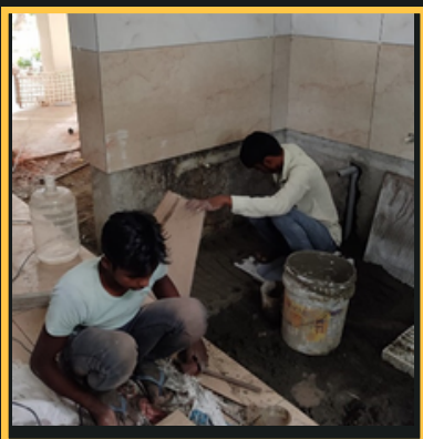
Laying tiles in restrooms
