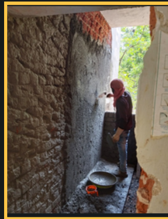
External and civil repair works
