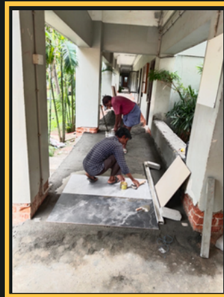
Laying granite flooring in the corridors
