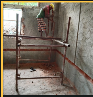
Making provisions for plumbing in restrooms
