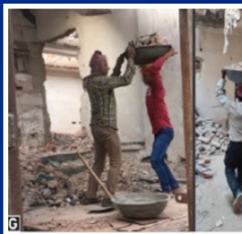
Process photos of deconstruction, material preparation and transportation
