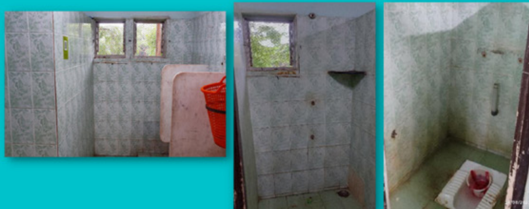
Before Dismantling work
