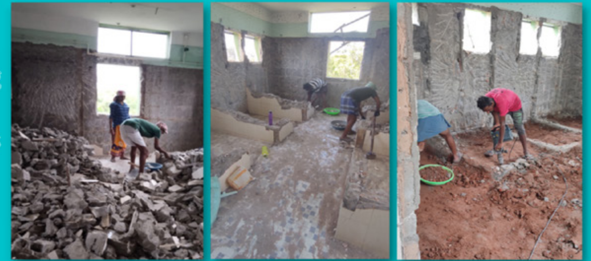
Dismantling work in progress
