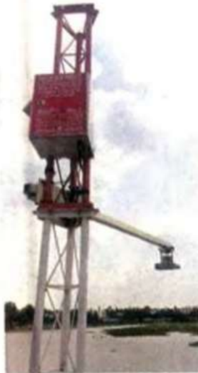
One of the flood monitoring systems installed by IIT-M
