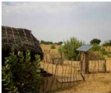
Solar panel installed at a village in India
